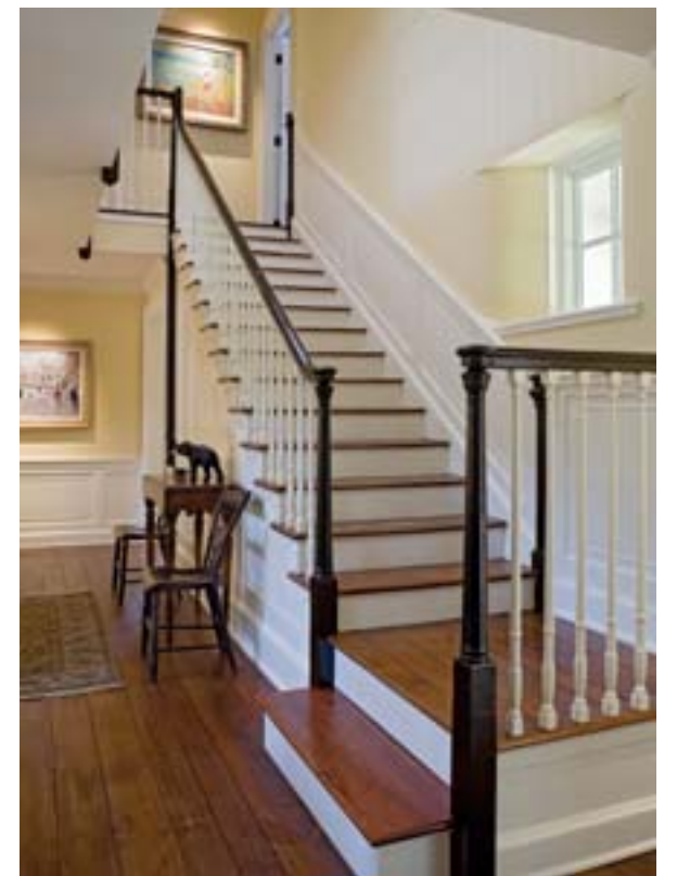
Below, right: New balusters, newel posts, and railings were incorporated in the antique staircase.
