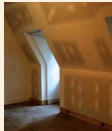
LEFT TO RIGHT: In one of the children's rooms, a false wall was built to disguise the duct-work. The far left photo shows the ducts attached to the wall; the center photos show the wall in various stages of completion. At far right, the new wall assembly is highlighted with a cheerful, contrasting paint scheme.
