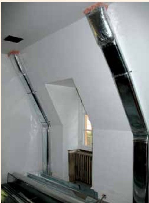
LEFT TO RIGHT: In one of the children's rooms, a false wall was built to disguise the duct-work. The far left photo shows the ducts attached to the wall; the center photos show the wall in various stages of completion. At far right, the new wall assembly is highlighted with a cheerful, contrasting paint scheme.
