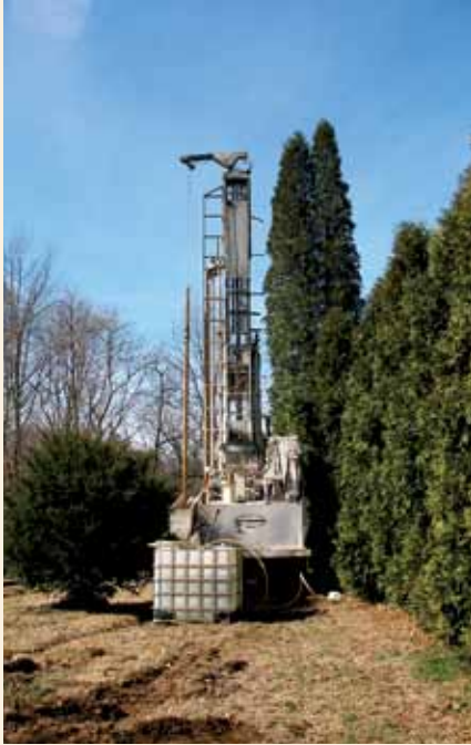
FROM LEFT: Installing the geothermal system first involved drilling six boreholes into the earth to access consistently warm temperatures. A trench between the bore field and the house holds both the refrigerant lines for the geothermal system and the electric wires for the solar array. Refrigerant lines in the attic run to the two separate units used to heat and cool the second and third floors.
