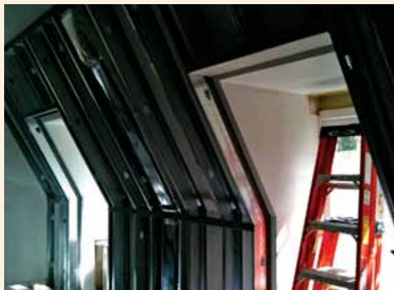
LEFT TO RIGHT: In one of the children's rooms, a false wall was built to disguise the duct-work. The far left photo shows the ducts attached to the wall; the center photos show the wall in various stages of completion. At far right, the new wall assembly is highlighted with a cheerful, contrasting paint scheme.
